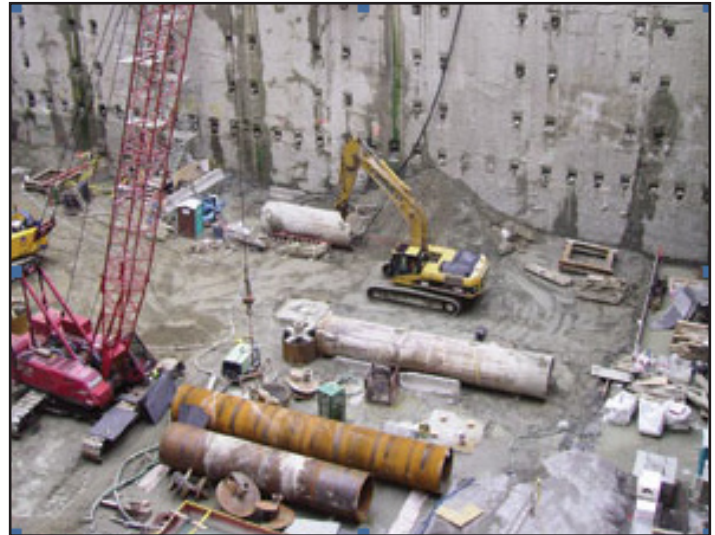
Photo: William J. Angelo/ENR Slurry wall and tiebacks protect tight site.
